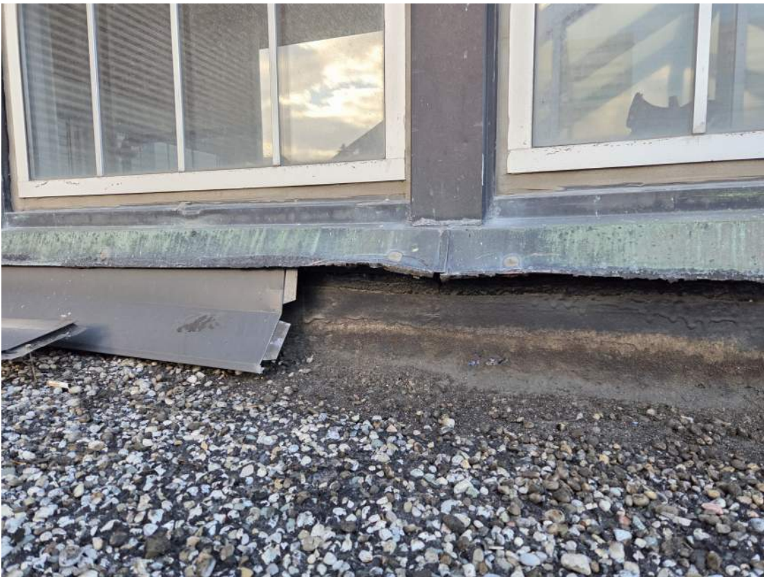
Existing metal flashing and copper sill at monitor roof to be demolished - See Demolition Note D10
