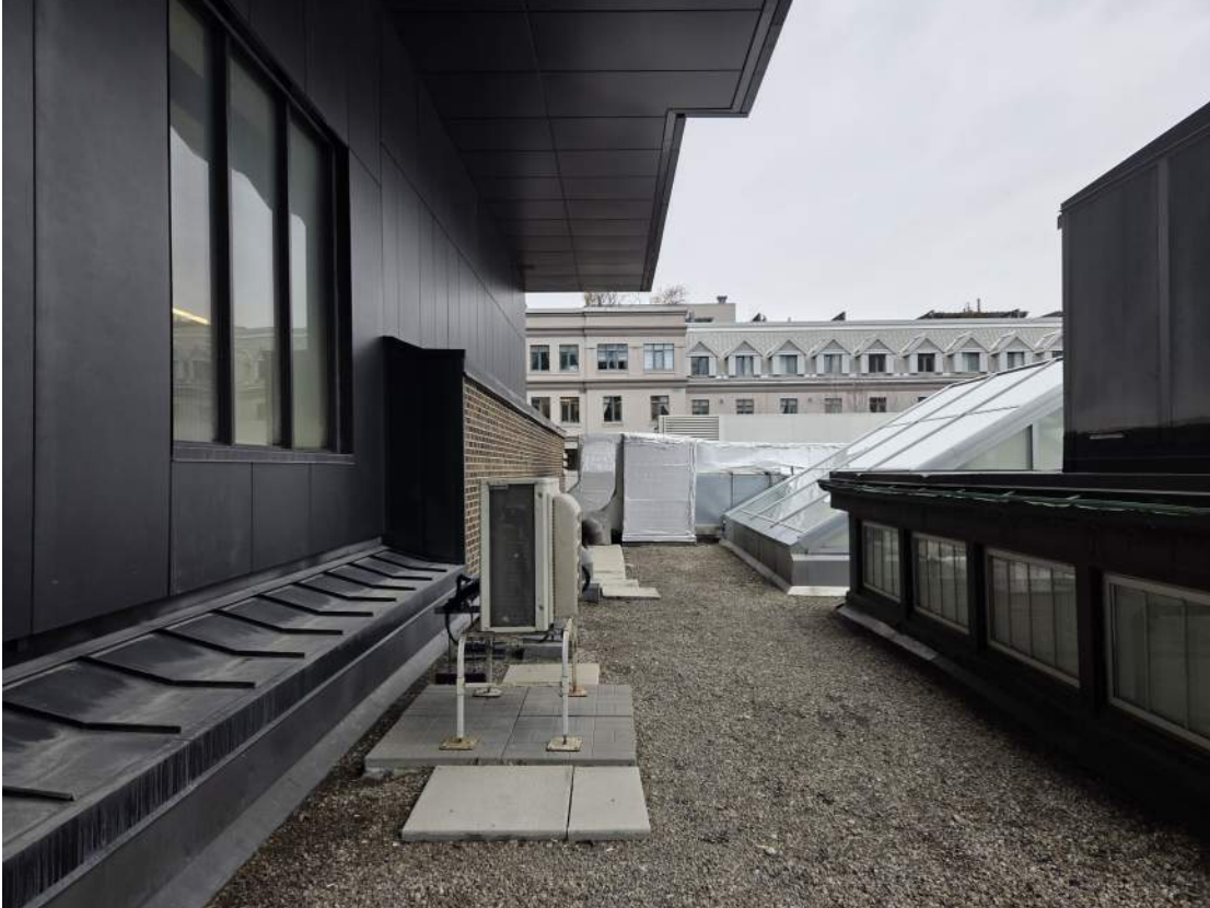
Existing metal flashing to be altered/replaced to accommodate new roof assembly - See Demolition Note D13
