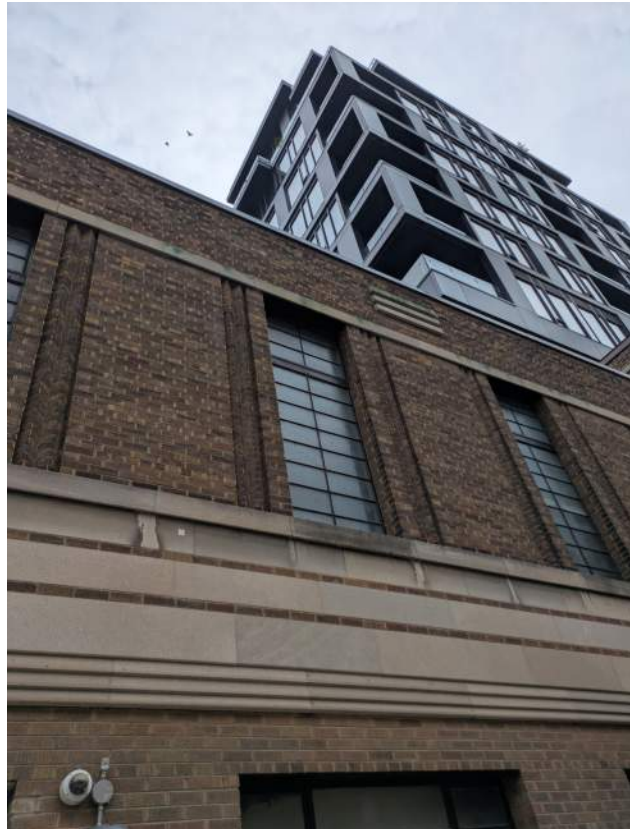
Existing exterior window sill to be repaired where necessary
