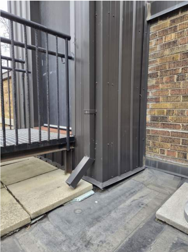
Existing metal siding to be removed and reinstated - See Demolition Note D11
