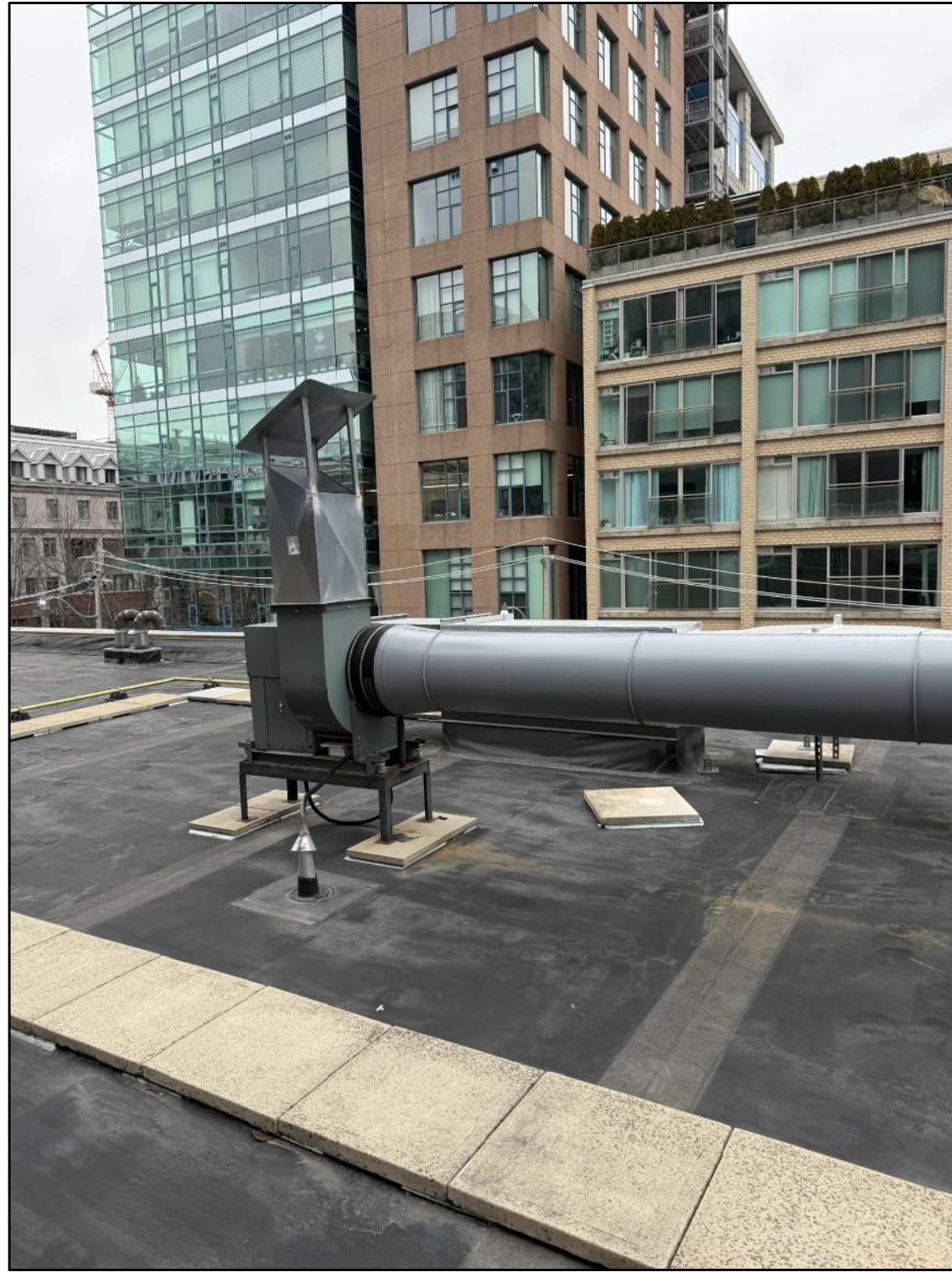
7 EXISTING KITCHEN EXHAUST FAN 'KEF-1' & KITCHEN DUCTWORK M5 SCALE: N.T.S.
