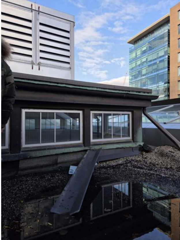
Existing gutters/rainwater leaders to be salvaged and reinstated - See Demolition Note D16
