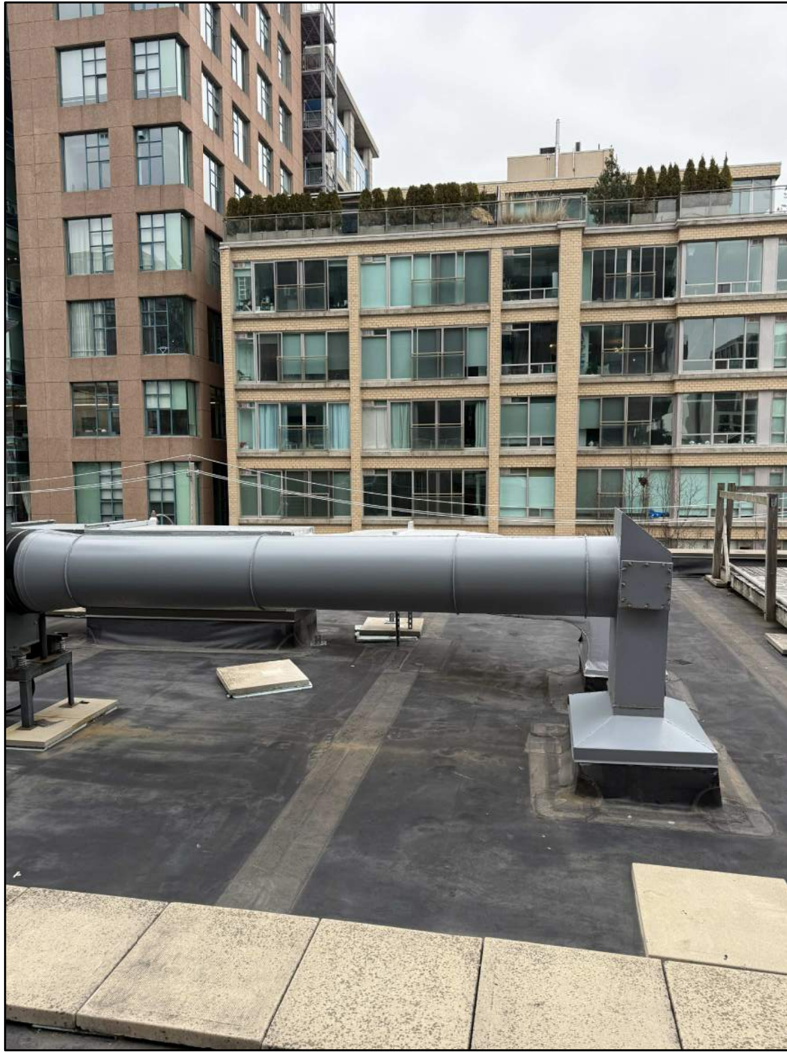
6 EXISTING KITCHEN EXHAUST FAN 'KEF-1' & KITCHEN DUCTWORK M5 SCALE: N.T.S.
