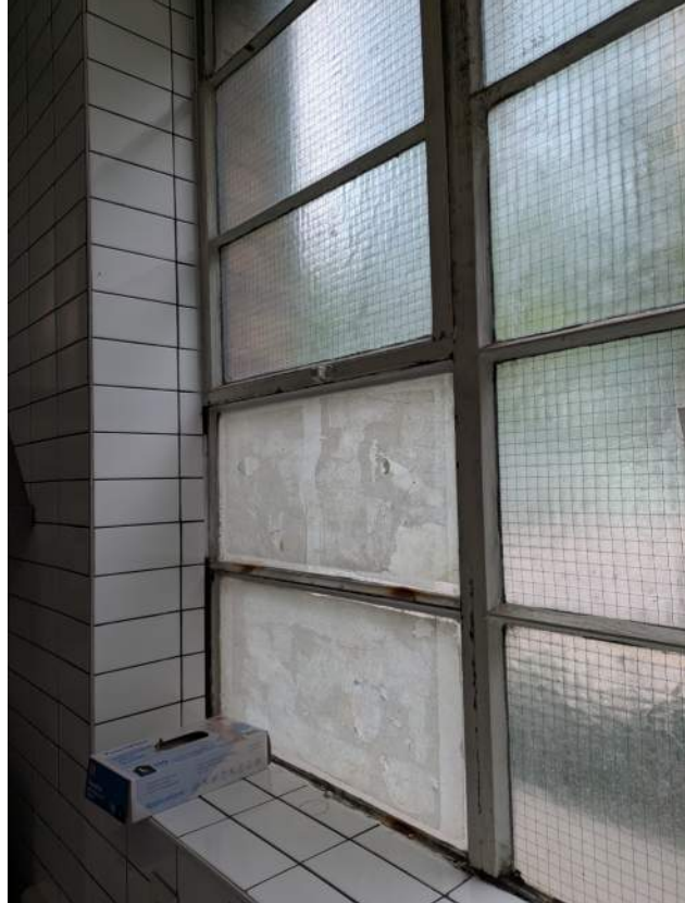
Existing window returns to be repaired where necessary
