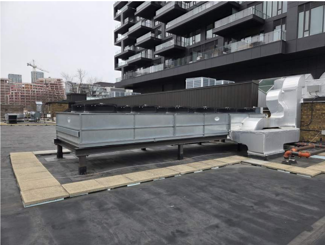
Fluid Cooler 'FC-1' to be relocated during roof replacement - See Demolition Note D2
