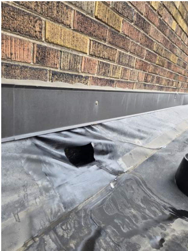
Existing metal flashing to be altered/replaced to accommodate new roof assembly - See Demolition Note D13
