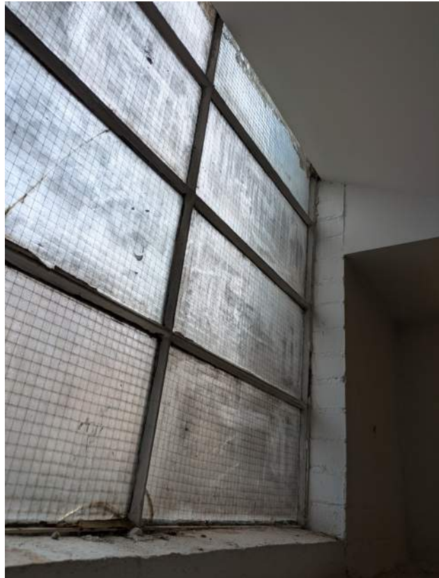
Existing masonry window sill and wall to be repaired and painted where necessary
