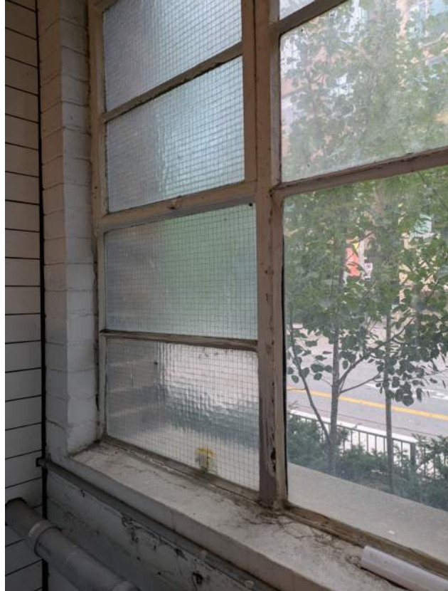
Existing masonry window sill and wall to be repaired and painted where necessary
