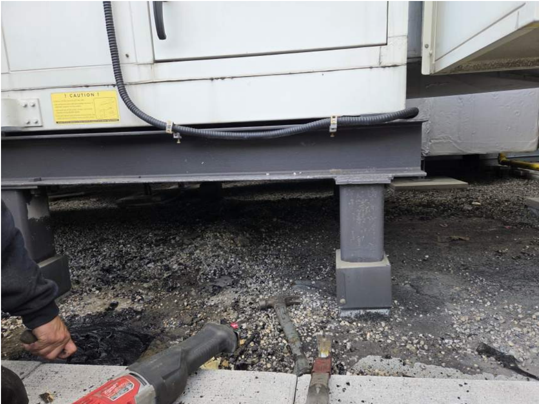
Existing membrane and flashing at structural support to be replaced - See Demolition Note D15
