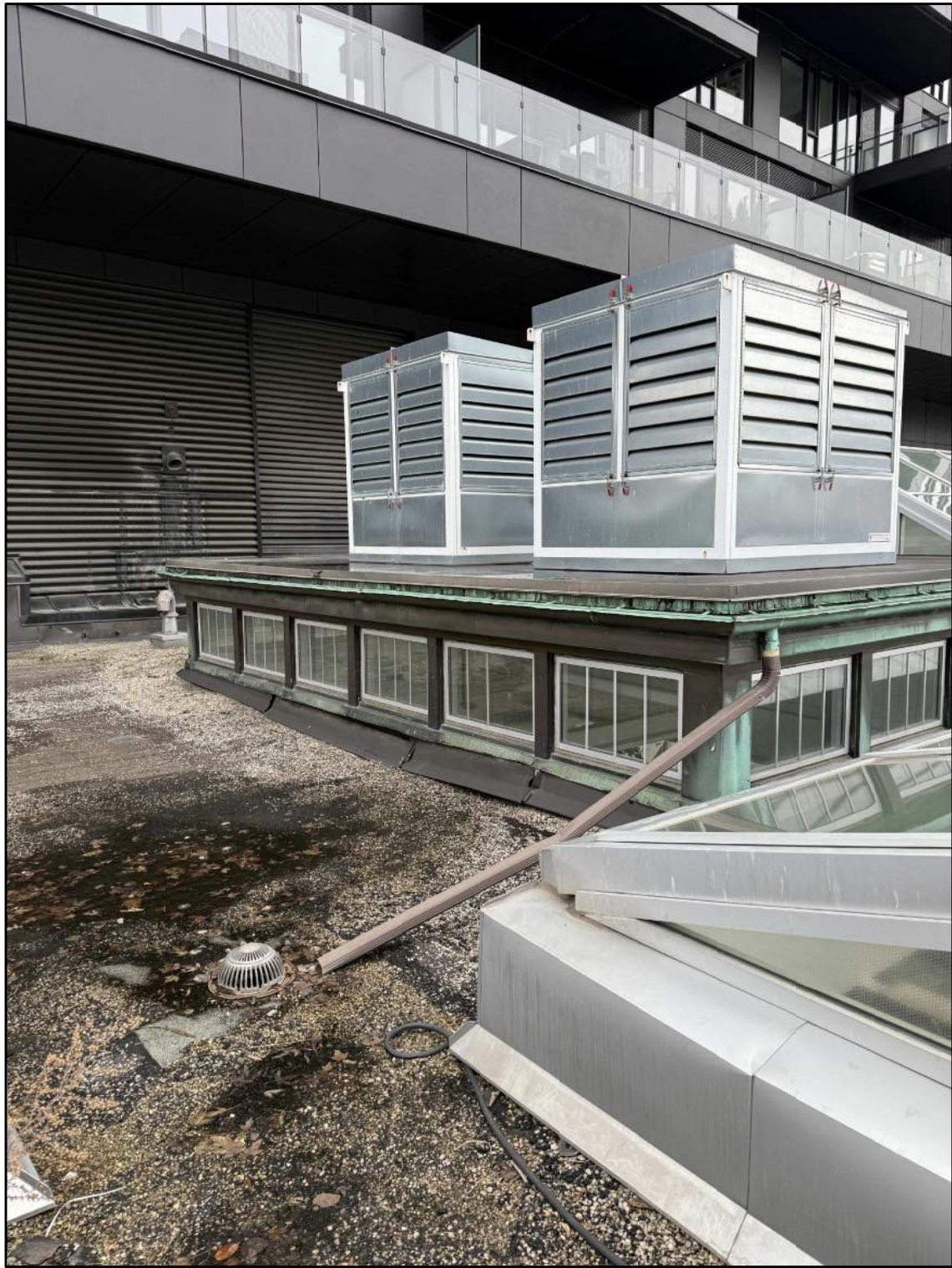
5 EXISTING ROOF DRAIN & SMOKE CONTROL EXHAUST FAN M4 SCALE: N.T.S.
