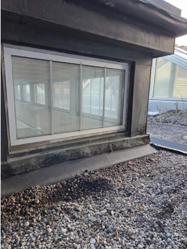
Existing metal flashing and copper sill at monitor roof to be demolished - See Demolition Note D10
