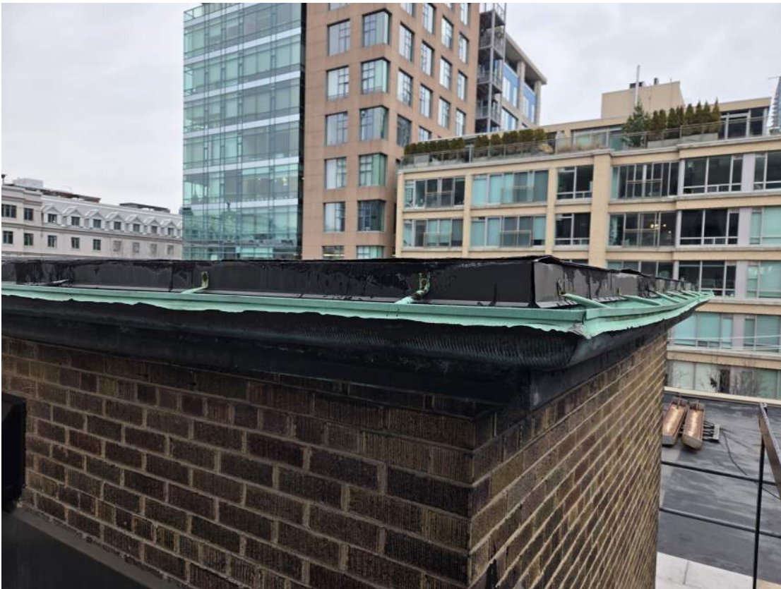
Existing gutters/rainwater leaders to be salvaged and reinstated - See Demolition Note D16
