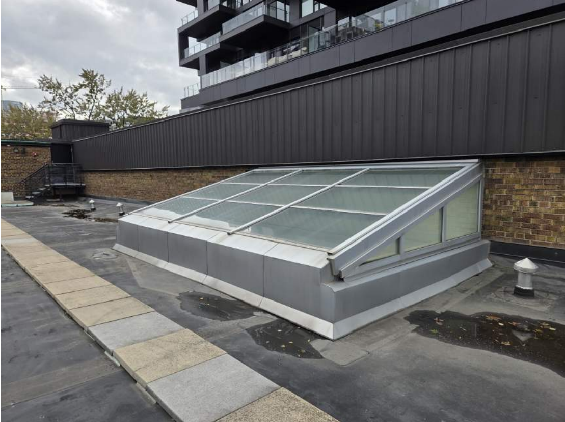
Existing break form aluminum at skylights to be replaced - See Demolition Note D6
