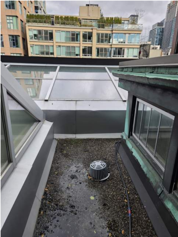
Existing break form aluminum at skylights to be replaced - See Demolition Note D6
