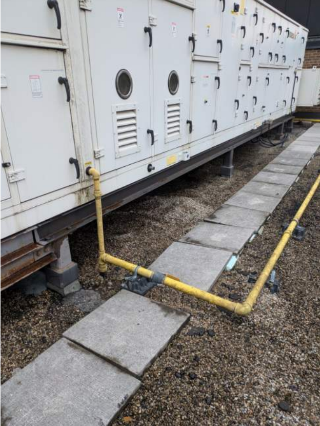
Fresh Air Unit 'ERV-1' to be relocated during roof replacement - See Demolition Note D2
