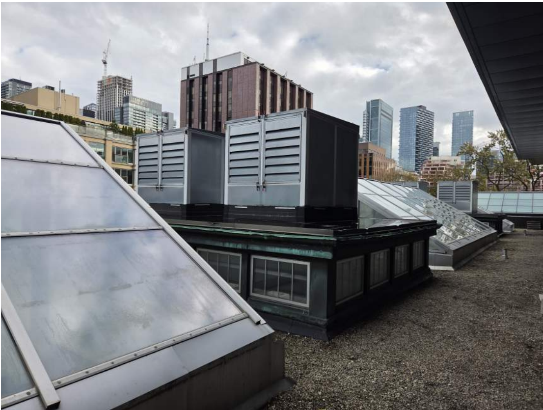
Existing doghouse for upblast fans to be removed and reinstated - See Demolition Note D9
